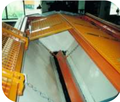
Aggregate sieve abrasive blast cleaned and relined with 3 coats of 209 EIP PU
