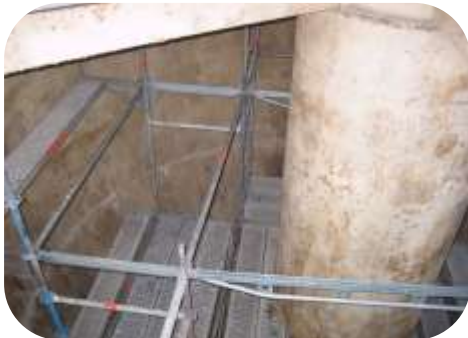
Chemical powder process vessel and chute were lined with 3mm of 209 EIP PU.
