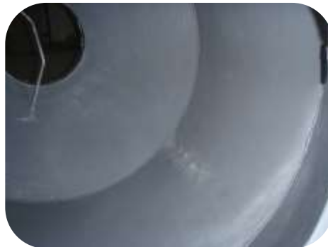
Process vessel operating at 95°C relined using 2 coats of 205 Ceramic HT
