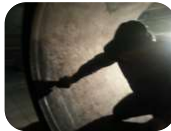
Process vessel required rebuilding and resurfacing. Internal substrates were mechanically abraded and relined using 202 Ceramic Repair Fluid
