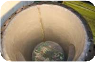
Sea water filter was in need of urgent repair. The internal surfaces were abrasive blast cleaned and lined with 2 coats of 202 Ceramic Repair Fluid. The coating was then post cured at 50C for 6 hrs to ensure the filter was back in operation within 24 hrs.
